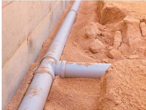
Figure 1.1.1 – Junction of plastic sewer pipes
